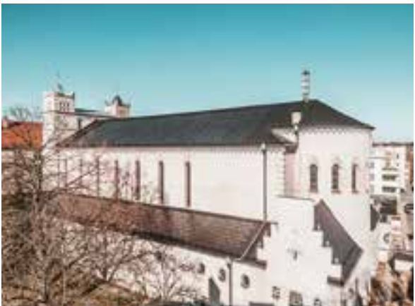
Object: Church St. Karl Borromäus Product: PREFA Solar roof tiles: 1,233 units, PREFA roof tile R.16 approx. 500 m² Power: 123 kWp, Cables laid: 4,600 m Roof area: approx. 800 m² Expected electricity production: 93 MWh/year Architecture: Architekturbüro Peter Troppmann Installer: Erhard Achtelstetter GmbH PREFA object consultant: Holger Voit Client: Kirchengemeinde St. Karl Borromäus
